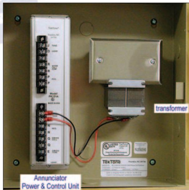
**3. The IH151NK includes a transformer and an annunciator power and control unit.**
